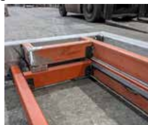
Inner edge beam return to door pocket
