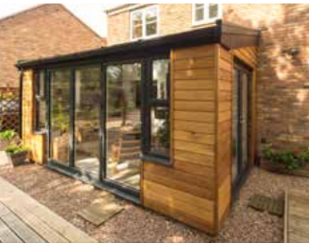
Horizontal Timber Boards
