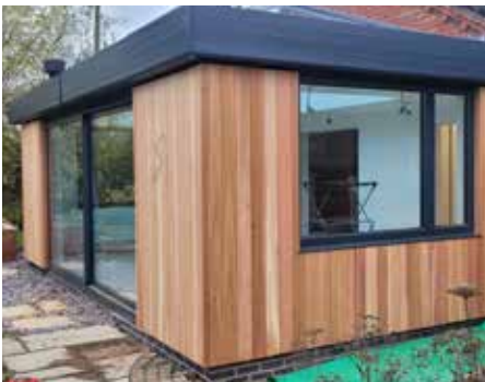
Vertical Timber Boards
