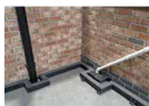
Intrusions for pipework
